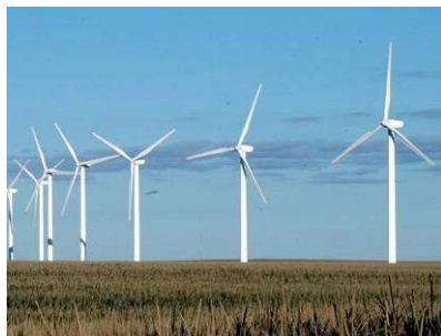
WIND POWER INSTALLATION VITERBO (Italy)
